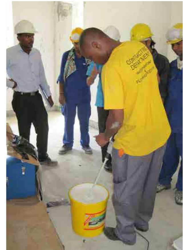
Training with Sikalastic 850W at the construction site
