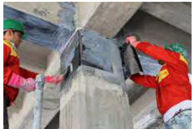
Sika Engineers training customers. This building was originally planned as a parking garage and now will be reused as a shopping center. Because of the different loads, for safety reasons many of the beams and columns were reinforced with SikaWrap. The built-up system is SikaWrap-230C with Sikadur®-330 impregnating resin, and Sikadur-31 for minor repairs and adjustments to the concrete substrate (prior to wrap application).
