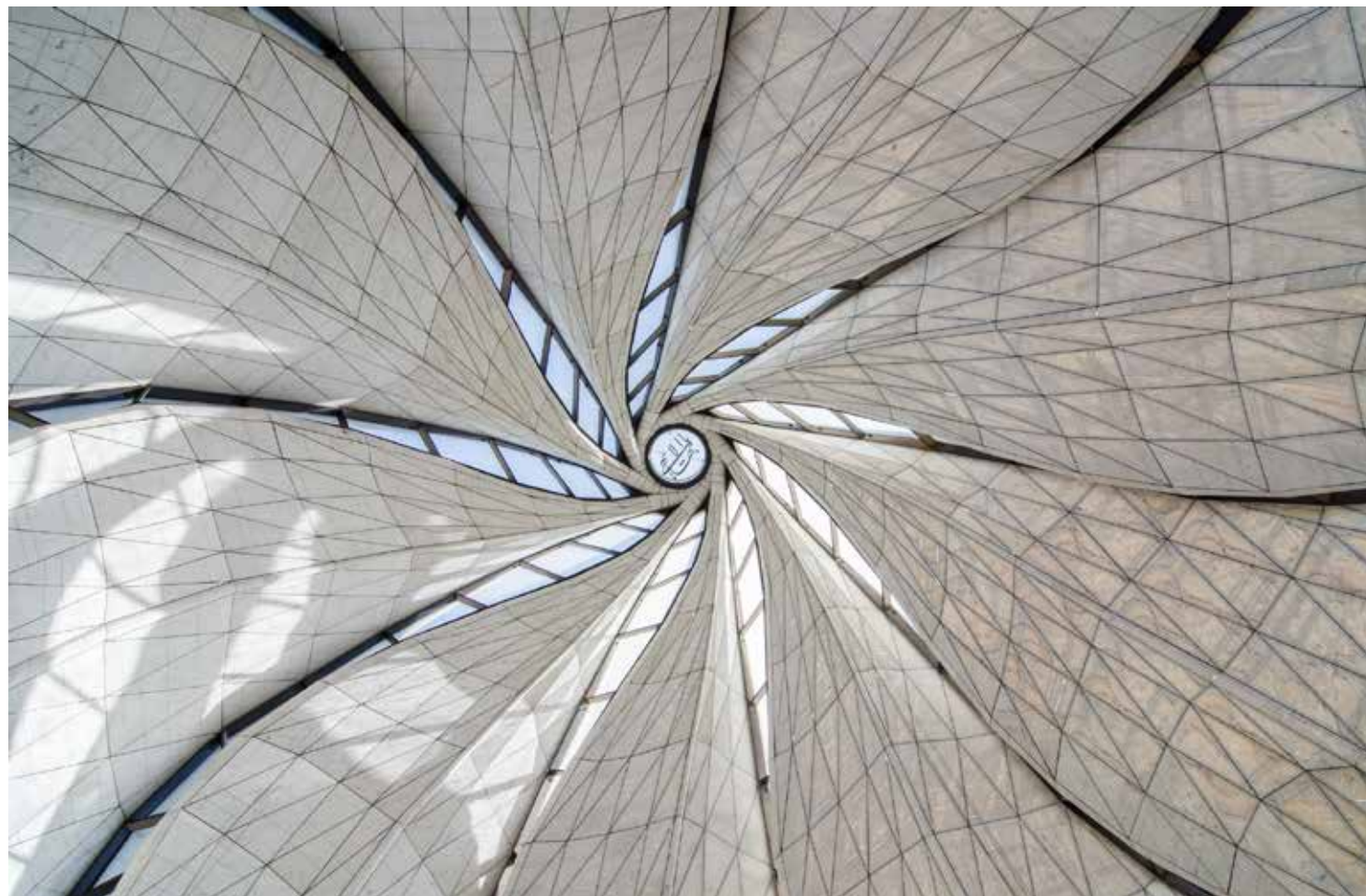
While the nine wings forming the temple are identical, each of them is formed by 3,000 unique elements of steel, marble and glass.
